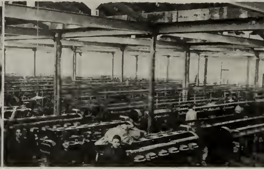
Erecting Whittin Machinery in Mill in North China
