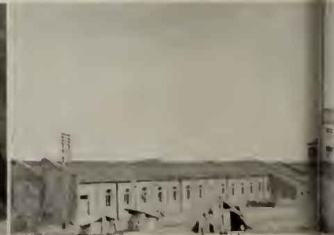
A view of the Hua Shing Mill
