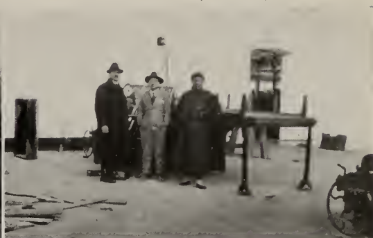
In the Picker Room, Hua Shing Mill
