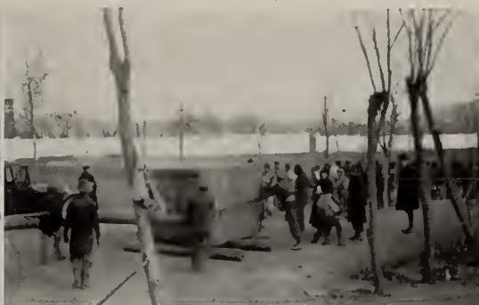
Manner of Transporting Whitin Machinery. This box weighed 6 tons. A rope was tied around the box and about fifty coolies dragged the box to mill. It took three days to drag the box one mile
