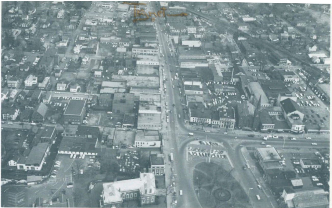
Air view of downtown Westfield looking north on Elm Street toward Westfield River. Athenaeum is in the bottom left center facing park. This is one of the finest public libraries in the state
