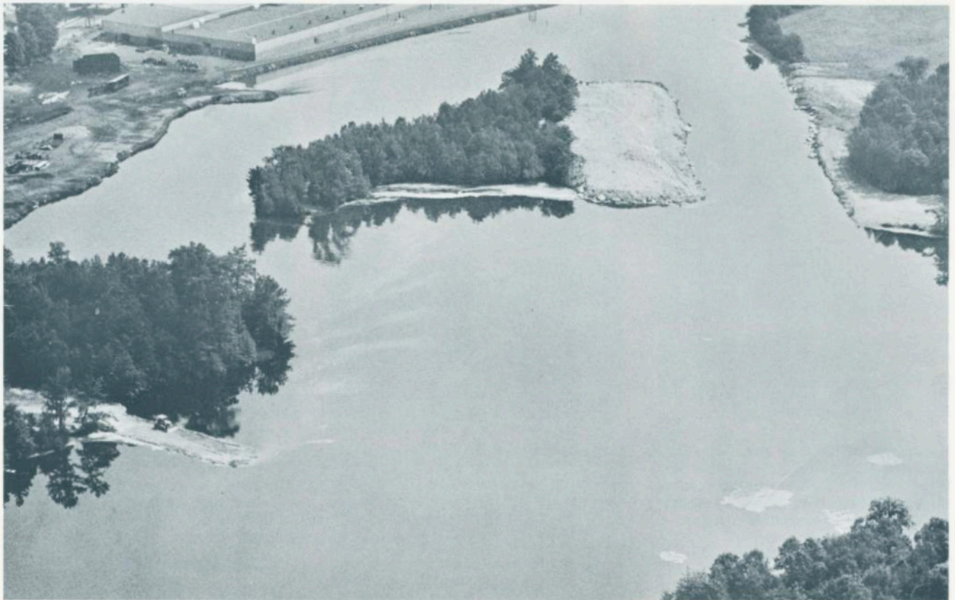
Pictured in the lower left hand corner of this photo is the start of the new earth dam which the Whitinsville Water Company is constructing across the lower south section of Meadow Pond. The dam will be 700 feet in length with a 100 foot spillway. It will extend from the peninsula on Main Street to the opposite bank where the gravel-packed well pumping station is located. The new dam will keep the Meadow Pond at a constant level, which in turn will hold up the water tables in the well fields that supply the town of Northbridge with drinking water. Furthermore, the dam will prevent the contaminated water of the Mumford River from flowing into the Meadow Pond. The completion of this project also will separate the drinking water reservoirs from the reservoirs whose water is used for power
