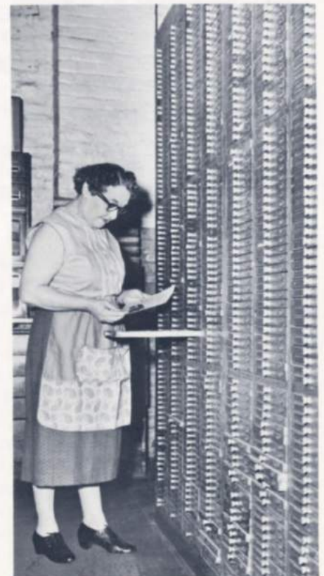
Every piece of type must be exactly .918" in height—with no tolerance whatever! Width and "body" size must also be checked
