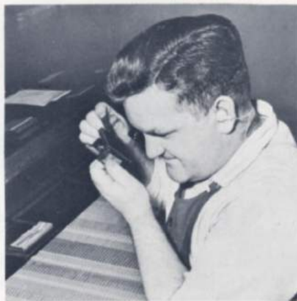
The letters are cast individually in the Barth casting machine. The single matrix is in the heart of the machine while a long row of single letters comes out like a ribbon at the lower right
