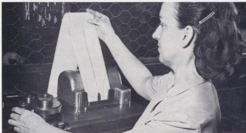
Louise O'Connell, departmental inspector on the Gear Job, making a pitch line chart of precision cut gears. Precision gears are individually tested for run-out on the pitch circle to insure smooth running which is an essential characteristic in machines producing fine textiles
