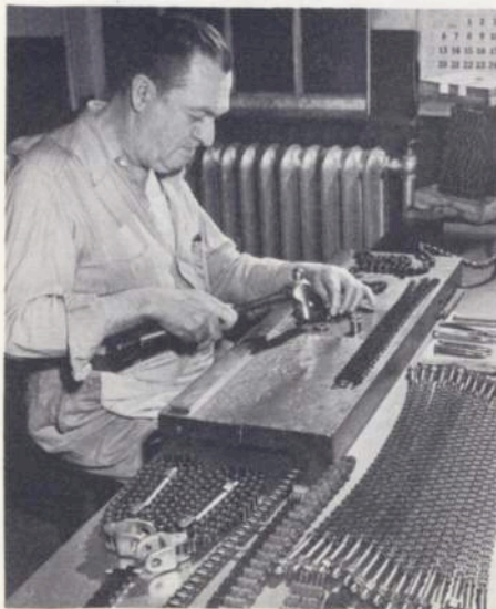
Above: Department 429, in addition to furnishing parts for the erecting floors, makes a number of complete assemblies. Here Mrs. Mabel Lemoine assembles a hank clock from the parts in the containers before her. Below: Francis Ledue is a specialist in the cutting and joining of chain. He is shown making up chain to the proper length for a builder motion on a spinning frame
