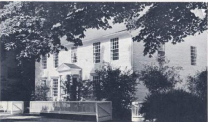
In the Webb House at Wethersfield, Connecticut, General Washington and the Count de Rochambeau planned the Yorktown campaign which ended the American Revolution. In each of the states many of the historic homes and public buildings are open to the public
