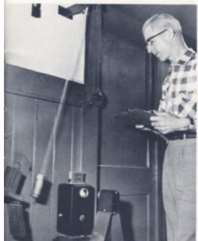
(Left): In many cases, the department designs and builds its own test equipment. Donald Benson uses a Whitin-built electronic Flexometer to test the flexibility of spindle driving tapes. (Center): At times, Department 575 has designed and built displays to assist the Advertising and Sales Departments. Bill Baron, left, and Assistant Supervisor James Youngsma examine a display they built for a textile exhibition. (Right): In their work, the department often must make or modify parts. Zigmont Mezynski, department machinist, is shown using a lathe for this purpose
