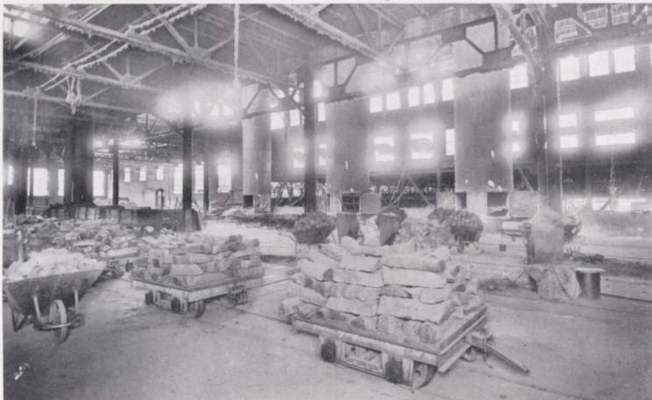
Charging Floor of Foundry
