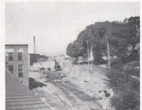
Excavation on the New Shop is Nearing Completion
