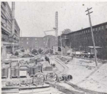
Progress on New Carpenter Shop
