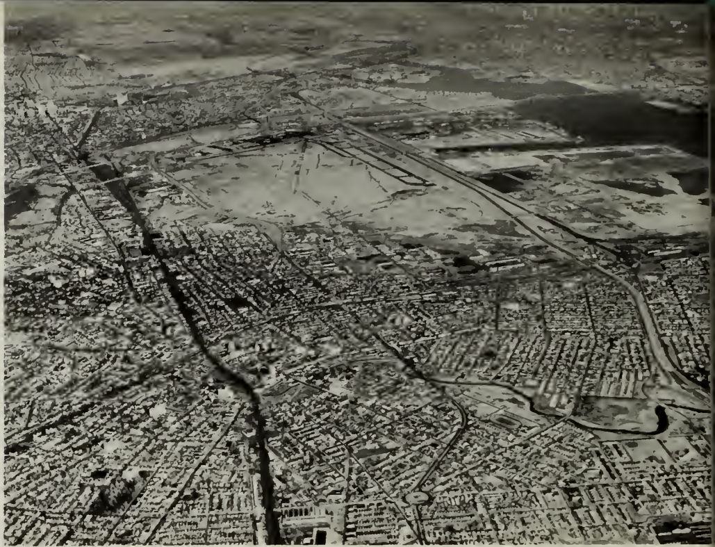
Nearness to New York which Elizabeth enjoys and profits from is demonstrated strikingly in this recent aerial photograph. The Central City is shown in the foreground, with downtown New York City nearby at right top. In between are Newark Airport, Elizabeth's one-time meadowlands where remarkable industrial growth is presently taking place, Port Elizabeth, on the Newark Bay. Pennsylvania and Jersey Central Railroad main lines cross in left center. U.S. Route 1 cuts a line through the city at center, the New Jersey Turnpike is seen at right and the Elizabeth River snakes its way to the Arthur Kill in the right foreground
