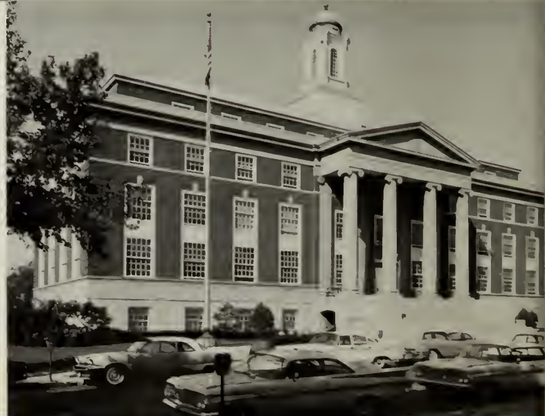
A clean City Hall is Elizabeth's boast. Built in 1940, this structure is noted as perhaps the best-maintained public building, with emphasis on cleanliness, in the state of New Jersey—or anywhere
