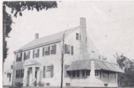
Newly Erected Home of William O. Aldrich, Manufacturing Superintendent of the Whitin Machine Works
