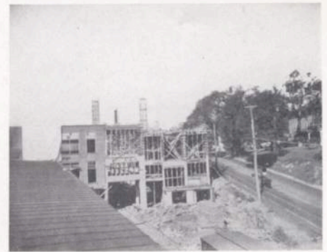
East end of new shop under construction
