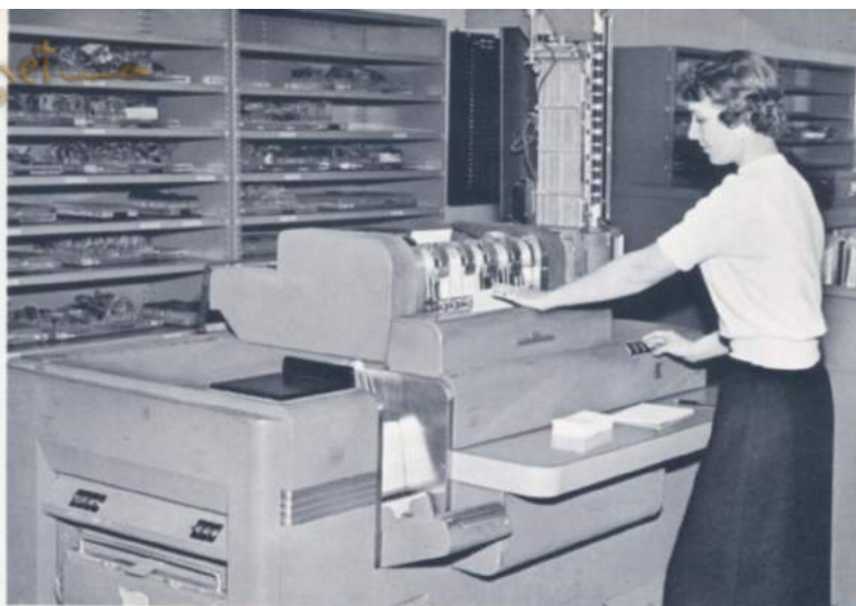
The actual printing of thirty-three hundred Whitin payroll checks a week takes a relatively short time on the IBM alphabetic subtraction machine which puts the amount on each check. This machine, operated by Christine Myott of Accounting, can handle 1800 checks an hour
