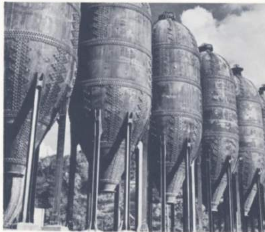
Above: From the chip storage bins, measured quantities of chips are poured into huge digesters, or cooking vessels. As much as 36 cords of wood may be processed in each digester in a single cook. Below: This line of digesters was photographed during the process of construction and before they were housed. In these digesters the chips are impregnated with chemicals and cooked under steam pressure to separate the cellulose fibers from the non-cellulose materials which bind the fibers together
