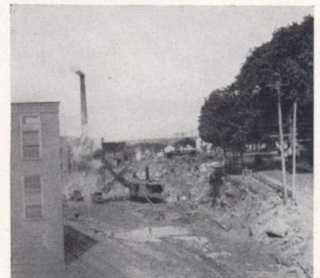
Progress on New Shop, June 14
