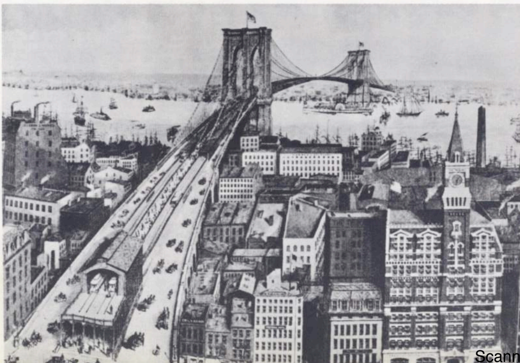
Soaring across the East River, the Brooklyn Bridge was opened to the public May 24, 1883. The 1595½ foot span, designed by John A. Roebling, was for twenty years the longest suspension bridge in the world
