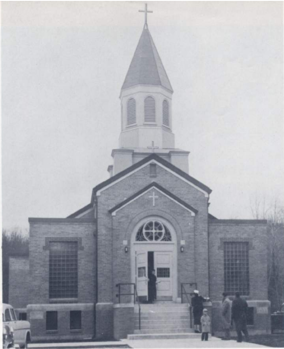
Soorp Asdvadsin Armenian Apostolic Church, built of brick along modified Byzantine lines, was erected over a period of three years at a cost of $100,000. It was consecrated on November 24, 1957
