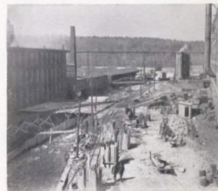
Site of New Carpenter Shop
