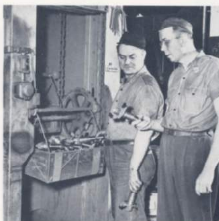
Bolster and case go through a degreasing process before final inspection. Leo Bouley unloads a basket as Dick Baker, supervisor, checks case for cleanliness
