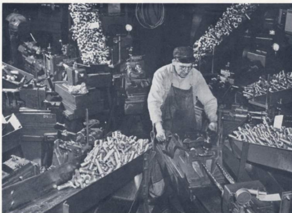
The first operation on a bolster case is the drilling of the lengthwise hole. Henry Gervais is shown starting one of the seven drills he uses to perform this operation
