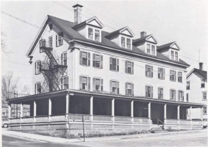
The Blue Eagle Annex, on Forest Street, once used as a boarding house to accommodate the unmarried among the Company's workmen, was razed in May. The space will be used as a parking area. The building is too old for further use. New quarters have been provided for the Plant Security Force and the Auxiliary Police who have been using the building for headquarters. The guards will occupy an area near the storeroom on the Comber floor and the Auxiliary Police will be located in a section of the stone building on Linwood Avenue near Research
