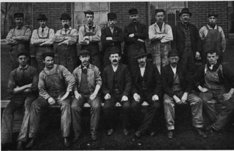
CARD ERECTING JOB OF 1895
