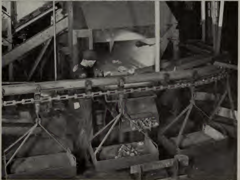
Top: Switchboard that controls the continuous molding unit. Once the switches are thrown to start the unit, the board controls the system automatically. Middle: Sand samples are taken about 20 times a day to our sand laboratory where they are checked for moisture content, permeability, and green strength. Bottom: Castings on their way to the Cast Iron Room after sand has been removed by shakeout machine
