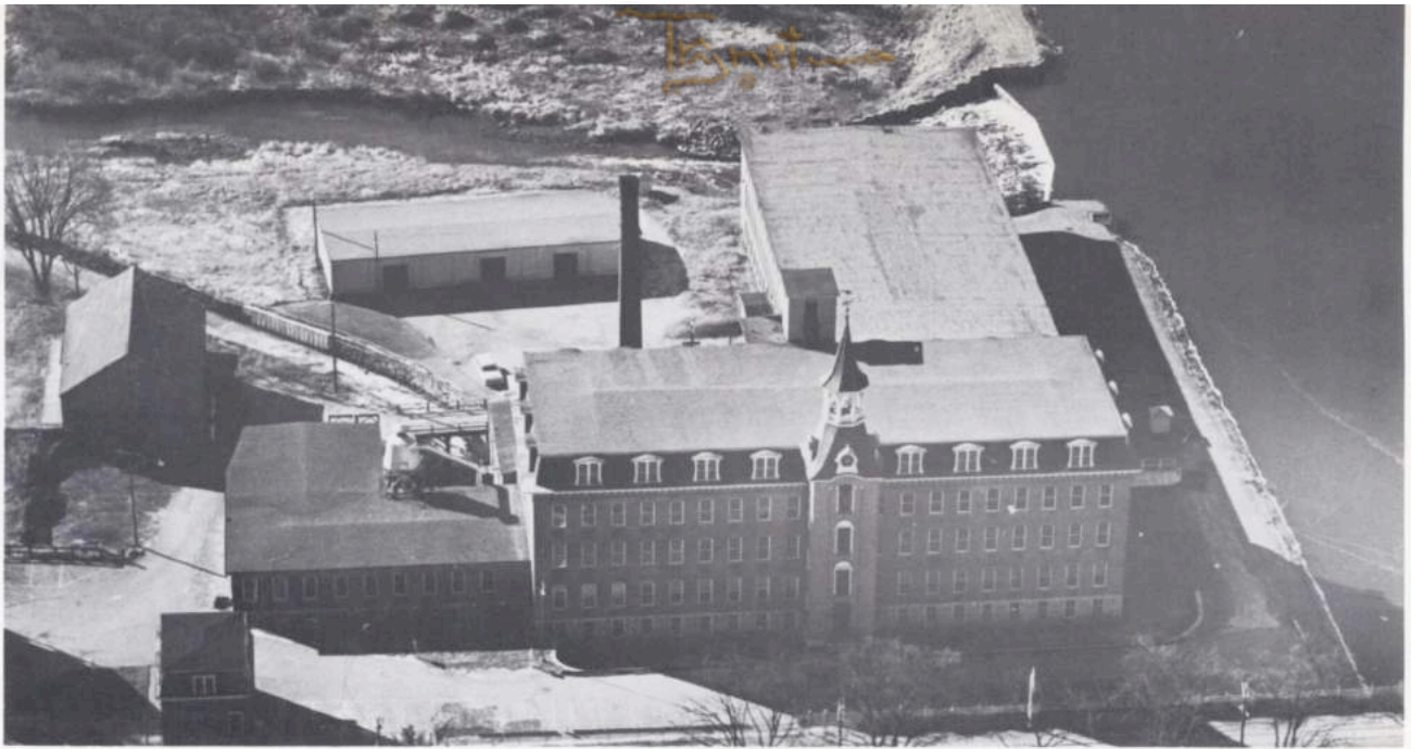
The Linwood Mill, used by the Whitin Machine Works for light manufacturing and storage until a few months ago, was sold to the Stylon Corporation, Milford, in December. In addition to its plant and headquarters in Milford, Stylon has plants in Florence, Alabama; Redondo Beach, California; and Salt Lake City, Utah. This aerial view shows the main mill, the office and two warehouses
