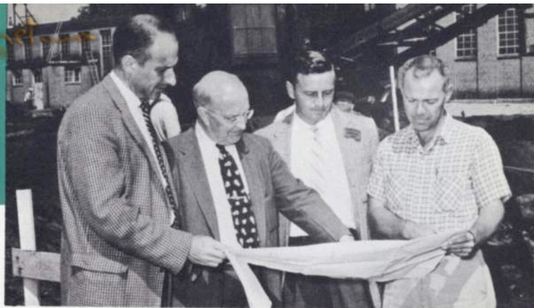
Representatives of Whitin and of the engineering firm check the foundation plans for the new manufacturing building No. 44. From the left, Mr. Edwin R. Davis, Asst. Maintenance Engineer in charge of construction of the new building; Mr. Philip B. Walker, Maintenance Engineer; Mr. Frederick Bacon, New England representative of the Luria Engineering Company; Mr. Allen S. Beck, Job Superintendent
