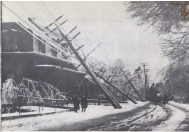
For three days—November 28, 29, 30—in 1921 the worst sleet storm in local history lashed at the Plant and the Town. Great damage was done to trees and power lines. Pictured is a section of Linwood Avenue
