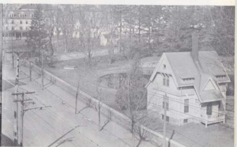
Where this house stood the Gymnasium was built in 1922. Here lived Grace Lowe, a teacher in Northbridge High School
