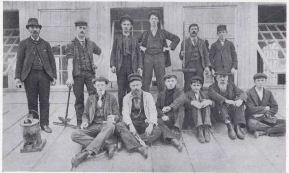
TIN JOB ABOUT 1895. PHOTOGRAPH TAKEN ON OLD FOUNDRY ROOF
