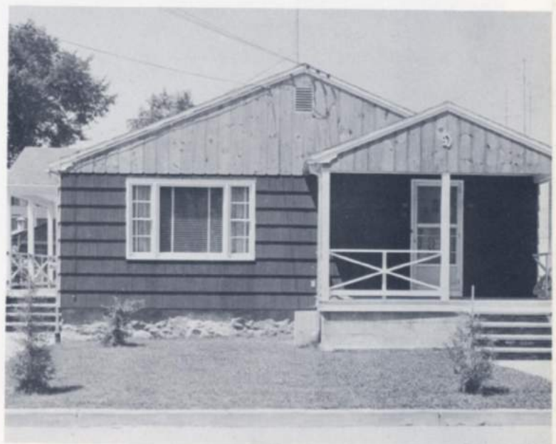
When the home of Corindo Debeneventura, Southbridge, was completely destroyed by the floods of Diane, the Red Cross built a new house for his family and in addition furnished it for them
