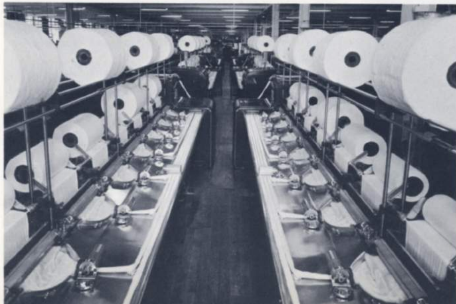
Two Bi-Coil drawn slivers emerge from the foot end of a Whitin Model J. Combed fibers such as these make finer, stronger, cleaner, more even, and more lustrous yarn when spun. These yarns are woven into fabrics for the highest-quality garments
