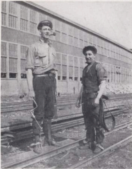
Mutt and Jeff, the Linemen
