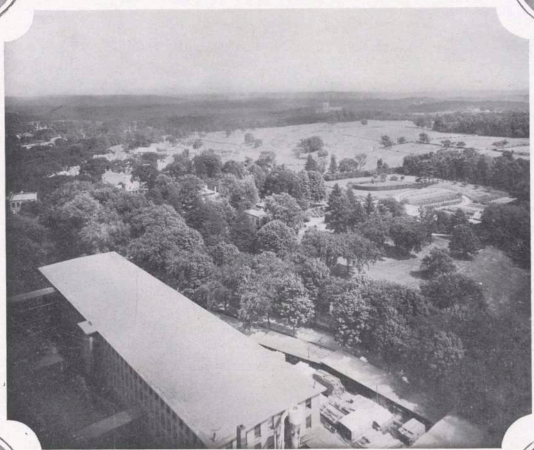
Whitinsville from the Air—View of No. 4 Carpenter Shop in Foreground
