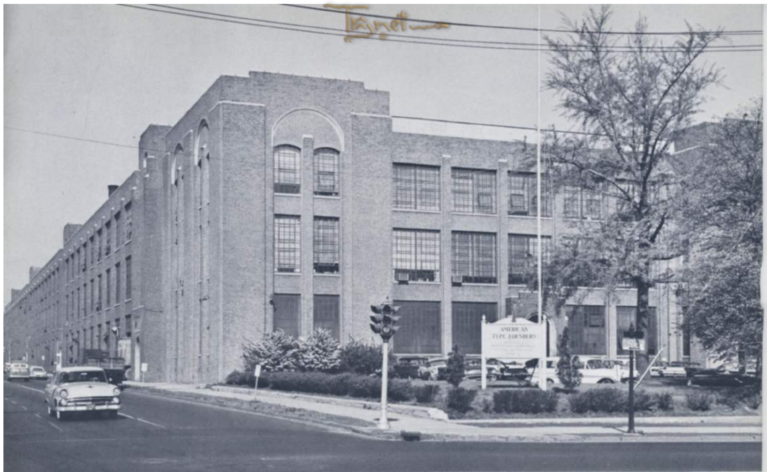
Building at 200 Elmora Avenue, Elizabeth, New Jersey, which houses the general offices and plant of American Type Founders, as well as the A.T.F. Type Foundry (largest in the world)
