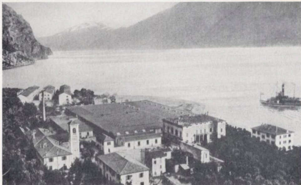
Campione Mill in Italy. Whitin Machinery now being installed
