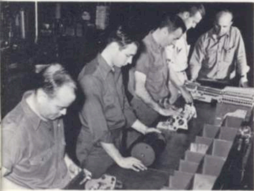
DUPLICATOR WORK now makes up a sizeable portion of the Whittin workload. This group is working on larger subassemblies, from the left: Francis Jacobs and an inker assembly, Roger Pouliot and a delivery cylinder, Ovila Gagnon and a water unit, Ernest Monsen and a jogger assembly. Joseph Gniadek, extreme right, is group leader
