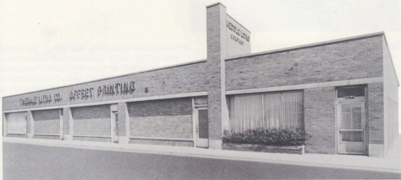
Fast-growing Tweddle Litho Company, St. Clair Shores, Michigan, now occupies entire 12,000 sq. ft. building in which it rented a single unit less than nine years ago. High-volume plant added 30,000 sq. ft. extension in September 1963, and installed a 36" ATF Web Offset Publications Press
