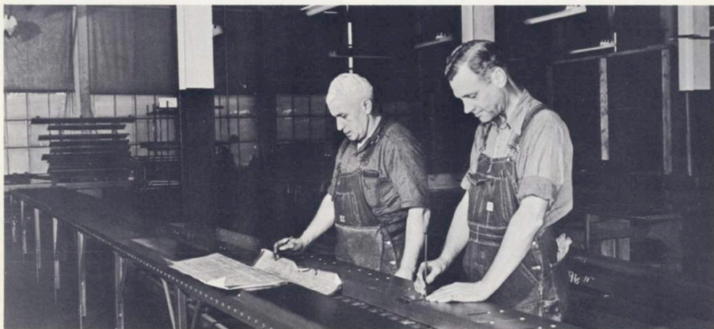
Precision is required from the initial step of laying out the roller beams. Here Romeo Gauthier, left, assisted by Henry Smith, checks his work against the blueprint
