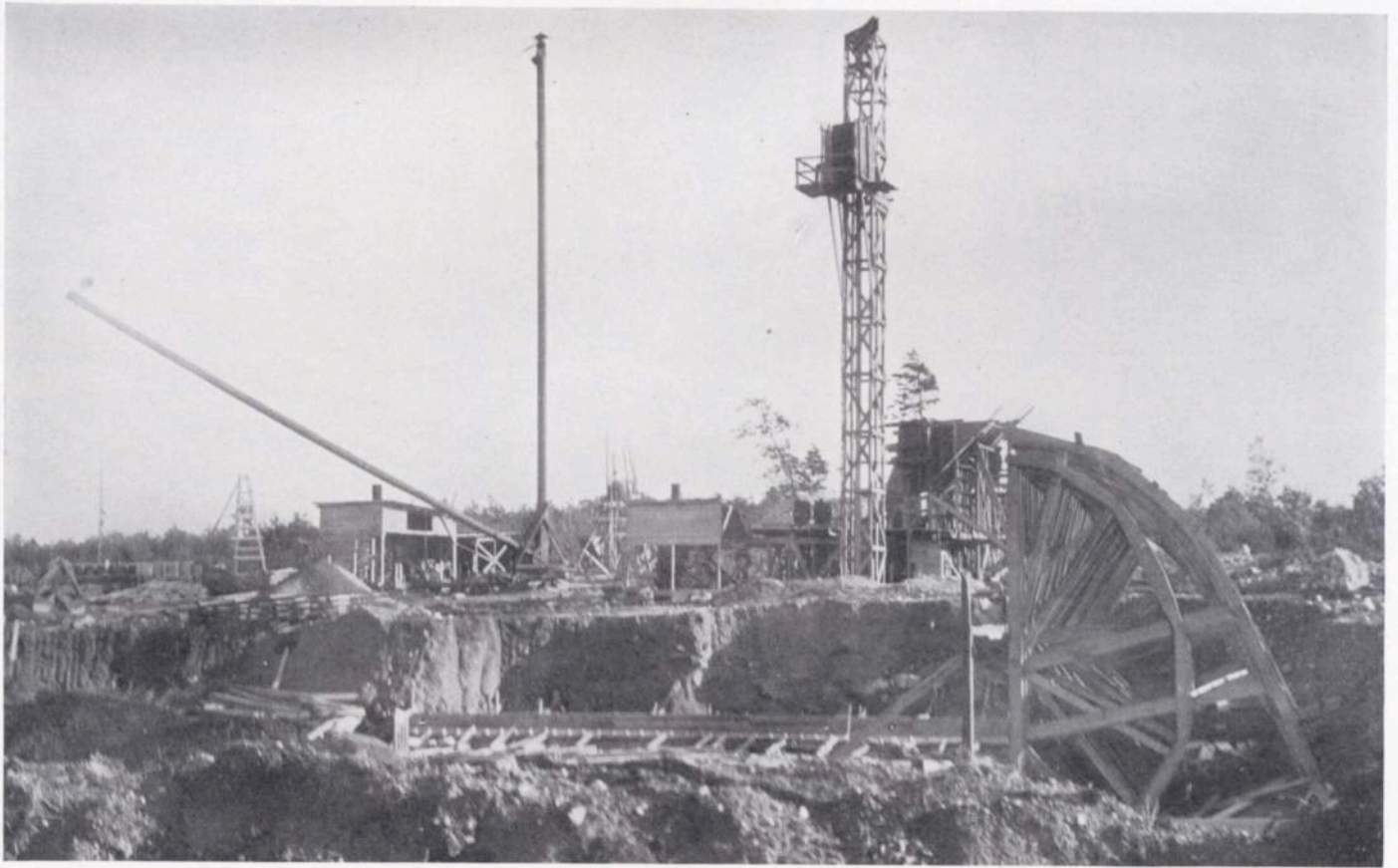
Constructing the Reservoir
